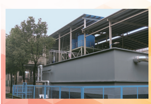
南昌工廠污水除磷設施 Facility for removing phosphate from sewage in Nanchang factory
